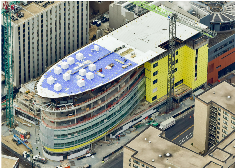
Aerial view of the Unisphere from the Northeast showing the Ground through 7th floors complete, Solar Tray structural steel framing erection nearly complete and curtain wall installation in progress (Dec. 2017)
