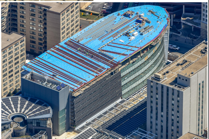
Aerial view of the Unisphere from the Southwest showing the primary structure essentially complete, solar panel installation at the Southern Solar Wall and Solar Roof above the parking deck in progress (Mar. 2018)
