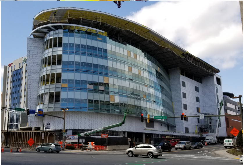
View of the Unisphere from the Northeast - concrete & structural steel Solar Tray complete, sloped curtain wall installation in progress. (Apr. 2018)
