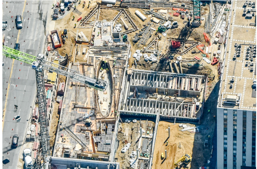
Aerial view of the Unisphere from the Southwest showing the Labyrinth partially complete, the Western portion of the Cellar in progress and the Eastern portion of the Ground floor form work (Apr. 2017)
