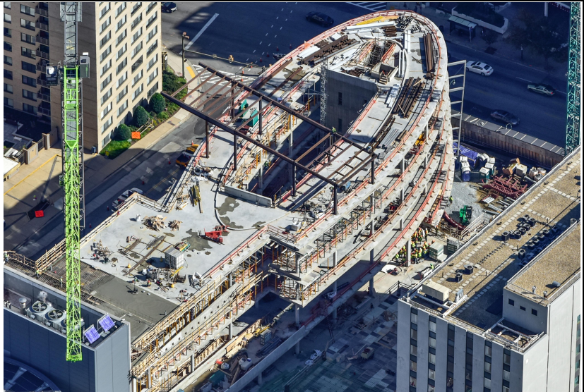
Aerial view of the Unisphere from the Southwest showing the Ground through 6th floors complete, 7th floor and Solar Tray structural steel framing erection in progress (Oct. 2017)
