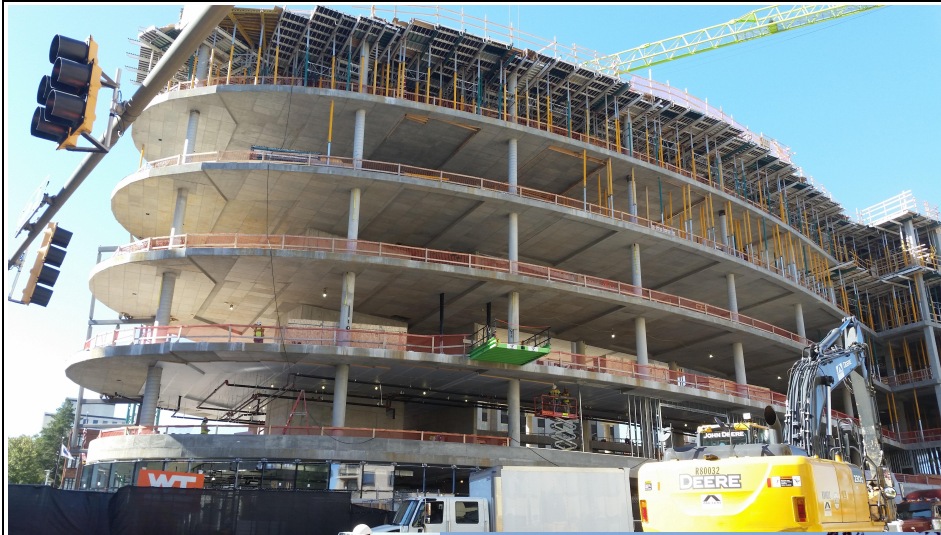
View of the Unisphere from the Northeast - Ground through 6th floors are complete, 7th floor is formed and shored. (Oct. 2017)
